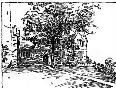
A CORNER OF THE NEW RESIDENTIAL HALLS FOR MEN
